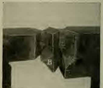
FIG. 3.—SHOWING A FILLER (B) INSERTED IN BROKEN LOCOMOTIVE FRAME.
